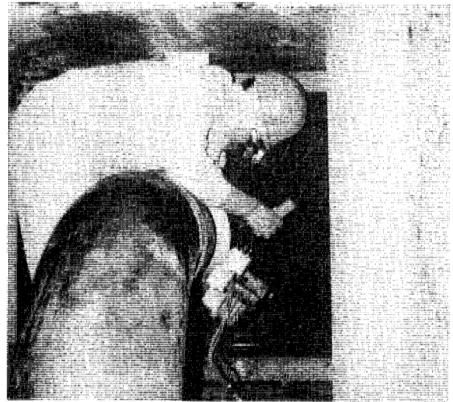
NDE contractor Marty Mingus running the "SAFT scanner" on a feedwater pipe at FitzPatrick.
